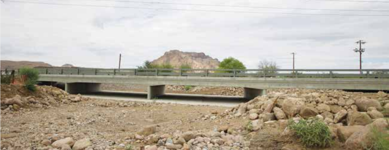
The new Panther Drive Bridge over the Queen Creek. Debbie Torres | CANP
