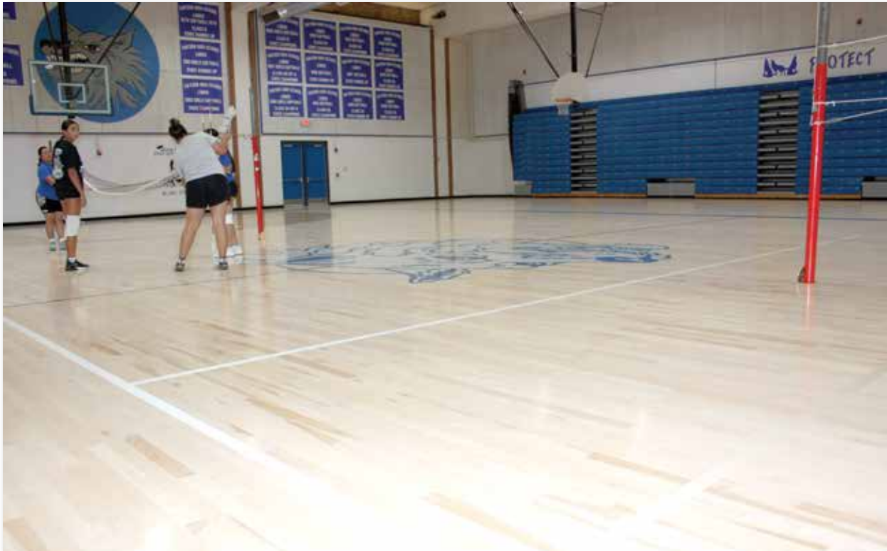
Girls attending the Volleyball Summer Camp at Hayden Schools were the first to play on the new gym floor. The new floor was installed over the summer.
