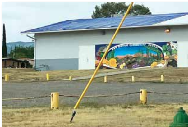
While the mess had been cleaned up, the roof atop the San Manuel Community Center was still covered with a tarp on Saturday. Lauren Carnes | CANP
